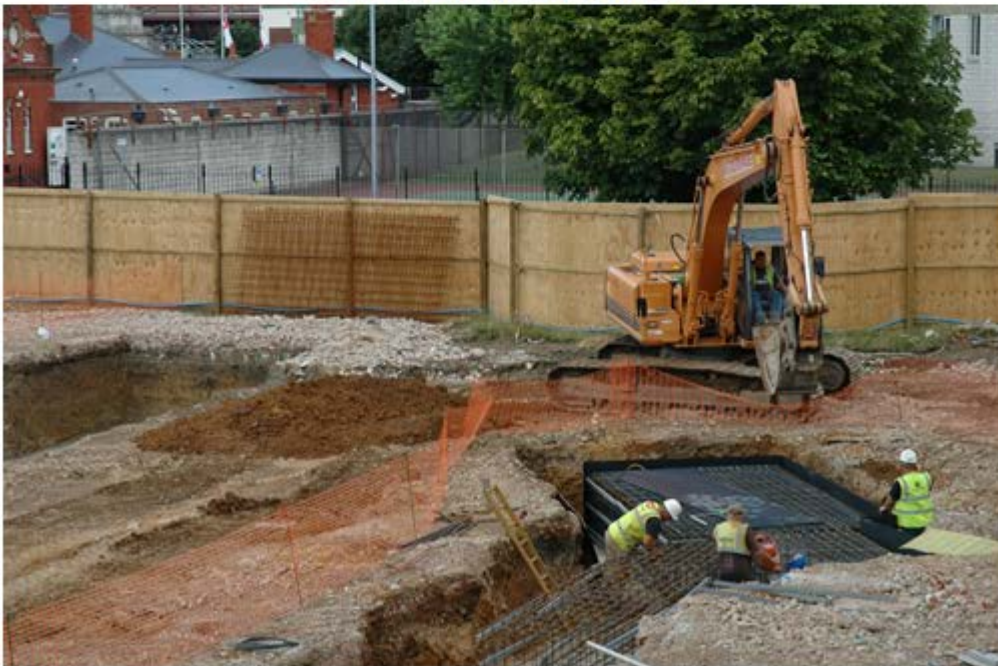
Assembling the reinforcing
