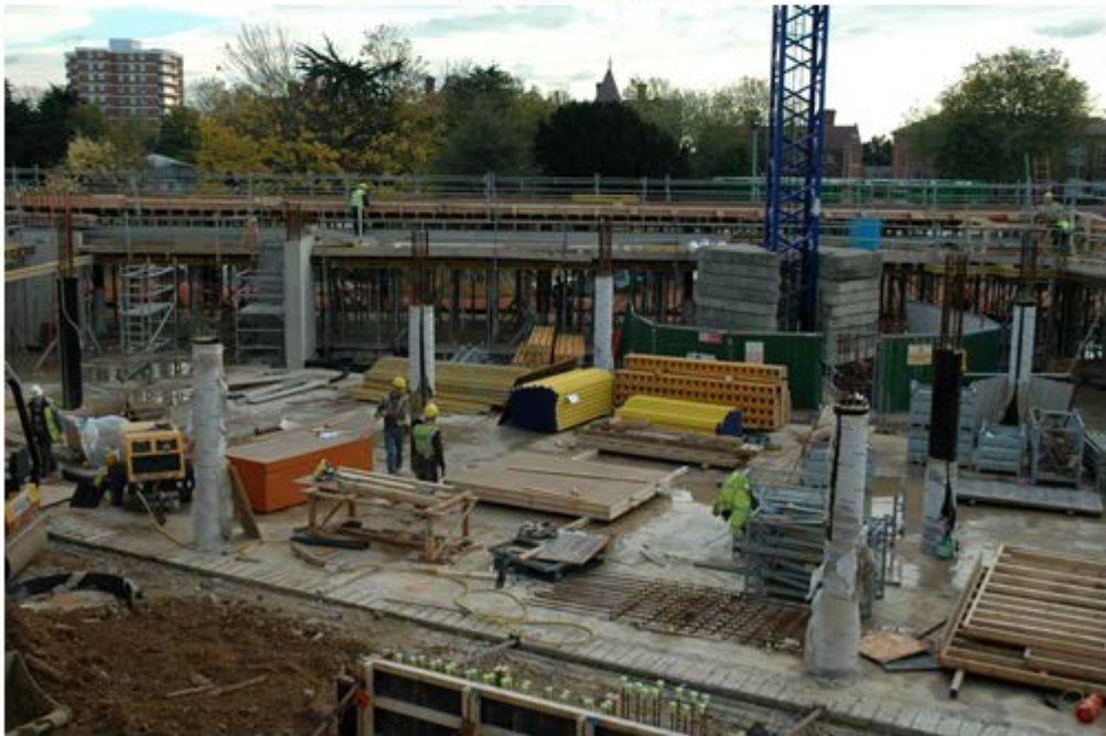
Assembling the shuttering
